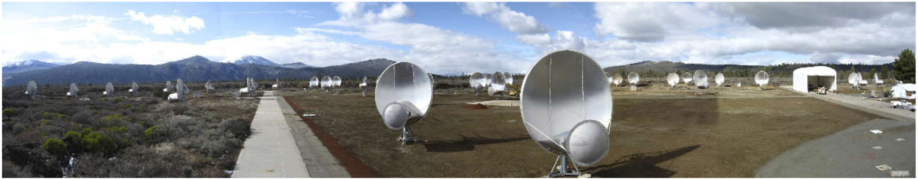
Figure 4: Allen Telescope Array 2000-2011. 42 antennas, with 4 simultaneous RF bands in the range 0.7 to 11 GHz. 4 100 MHz bandwidth, 1000 channel correlators, 3 beamformers. Used for radio surveys, HI in spiral galaxies, radio transient surveys, SETI.
