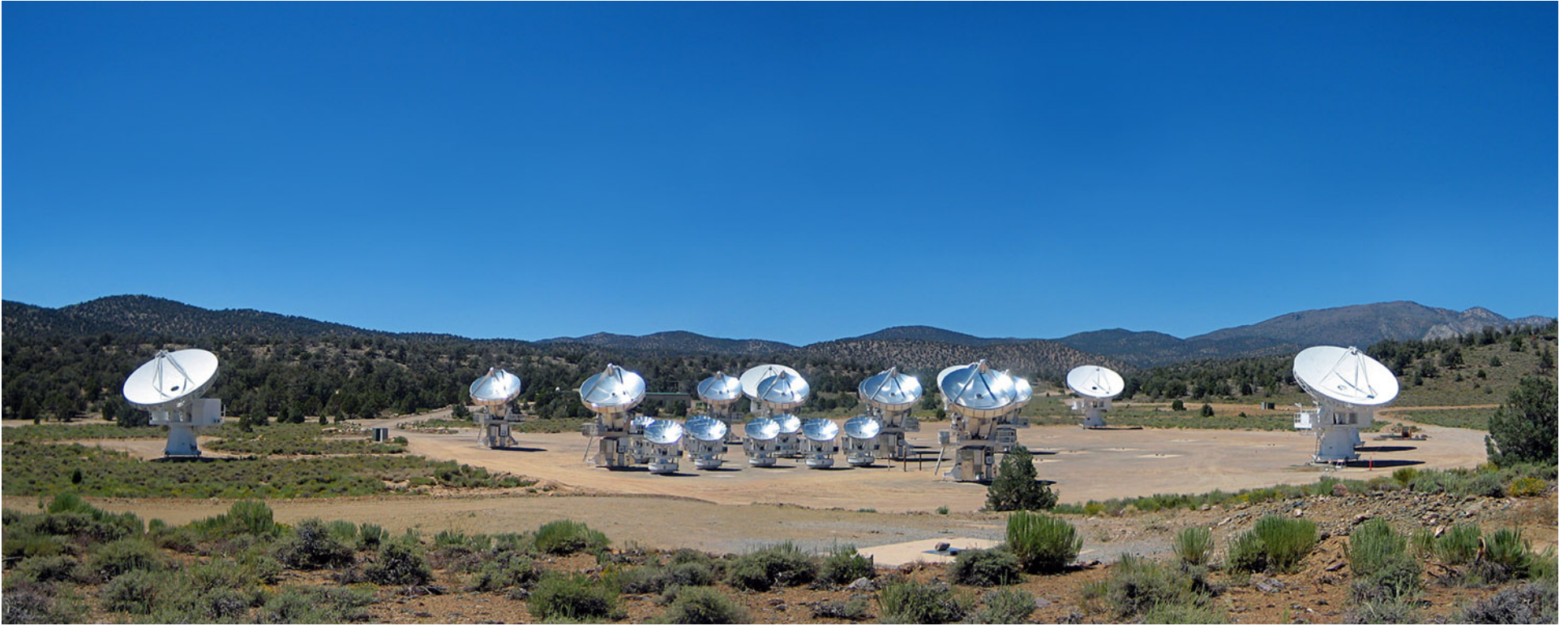
Figure 6: The CARMA 23-element interferometer at Cedar Flat. Heterogeneous array with six 10 m, nine 6 m, and eight 3.5 m antennas providing projected antenna spacings from 3.5 m to 2 km. Receivers at 1cm, 3mm, and 1.3 mm. 4 GHz bandwidth correlator providing 16 spectral windows. Used for imaging star formation regions, galaxies, planets, protoplanetary disks, molecular clouds, galaxy clusters. Recent 1.3 mm VLBI using telescopes in Arizona, California and Hawaii with phased arrays at CARMA and SMA detected 30 microarcsec structure in the 4 million solar mass Black hole at the Galactic center.
