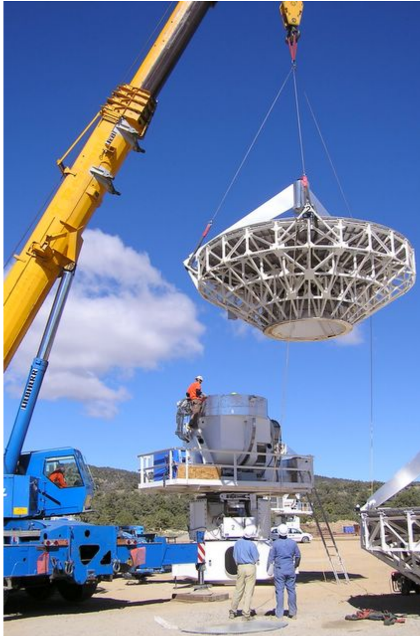
Figure 13: Re-building 6m antennas at CARMA
