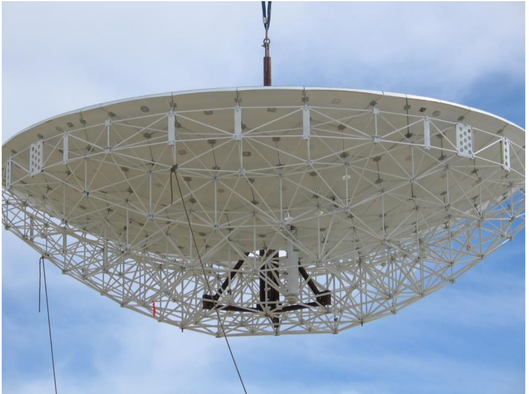
Figure 16: Re-building 10m antennas at CARMA
